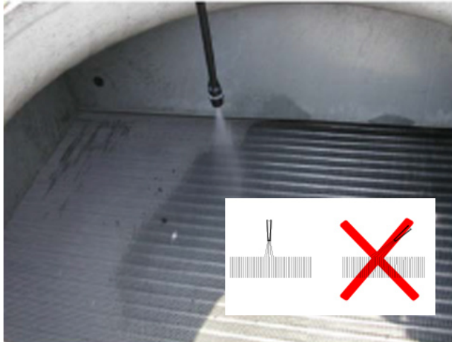
Figure 43: Allowed angle of low pressure cleaning water jet against coil material
